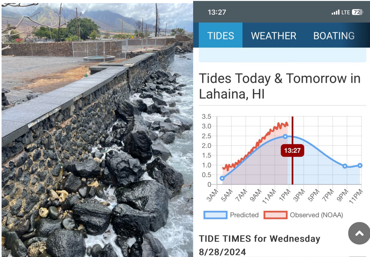
Figure 5- Transect #816 Seawall During King Tide (6 inches above normal)
